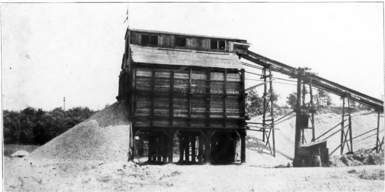
Conveyor to Sizing Screens. Note Storage Bins and arrangement for Loading Trucks
